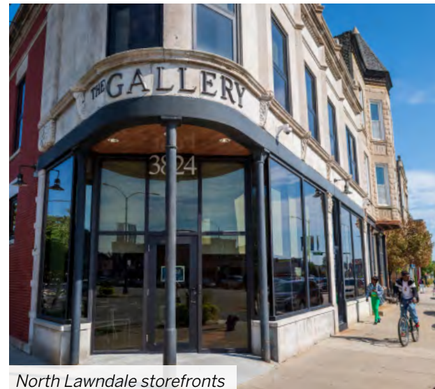
Recently opened restaurant in North Lawndale
