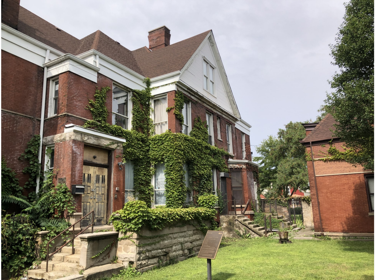
Looking northwest at the main house. The altered coach house is at right.
