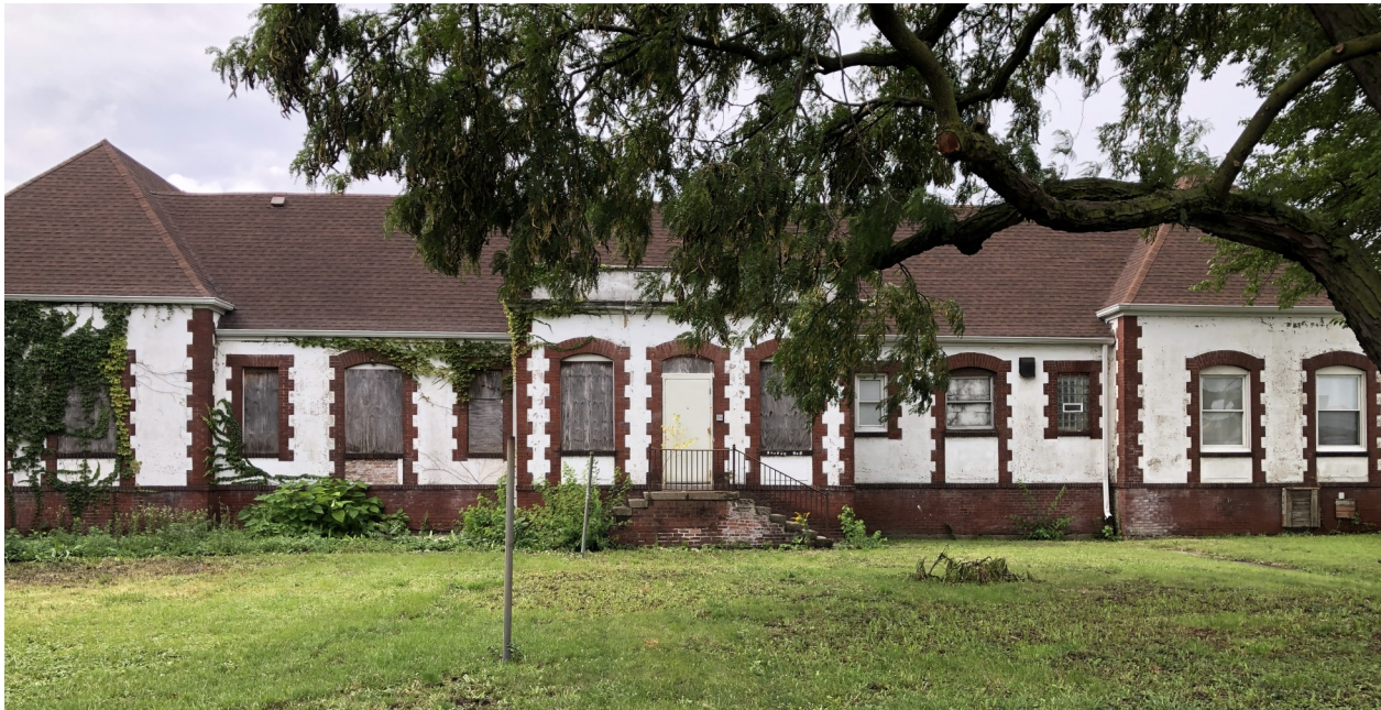
The east elevation of the dormitory.
