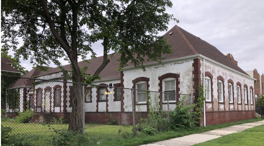
The dormitory at 2678 West Washington Boulevard.
