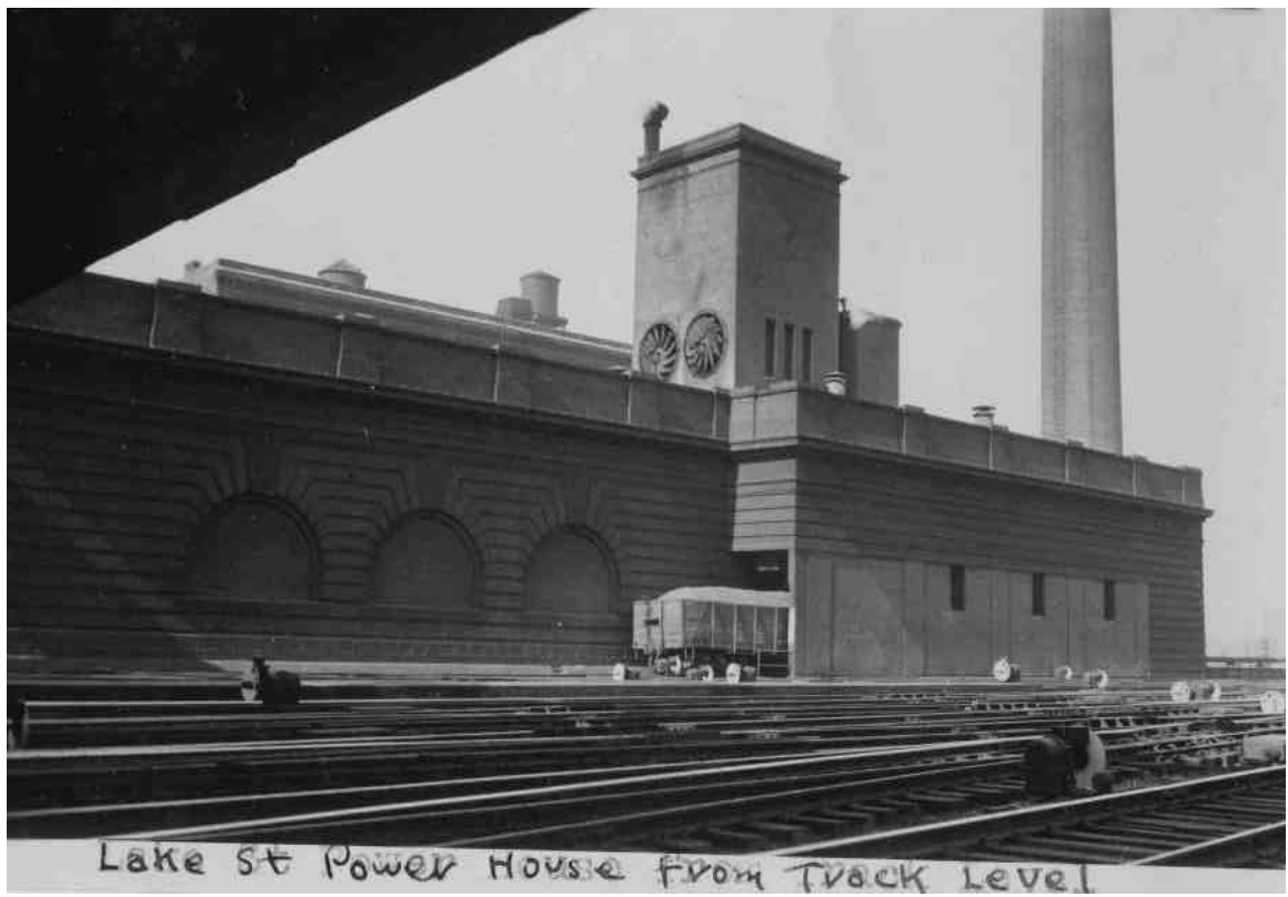
Historic views of the Chicago & North Western Railway Powerhouse.
