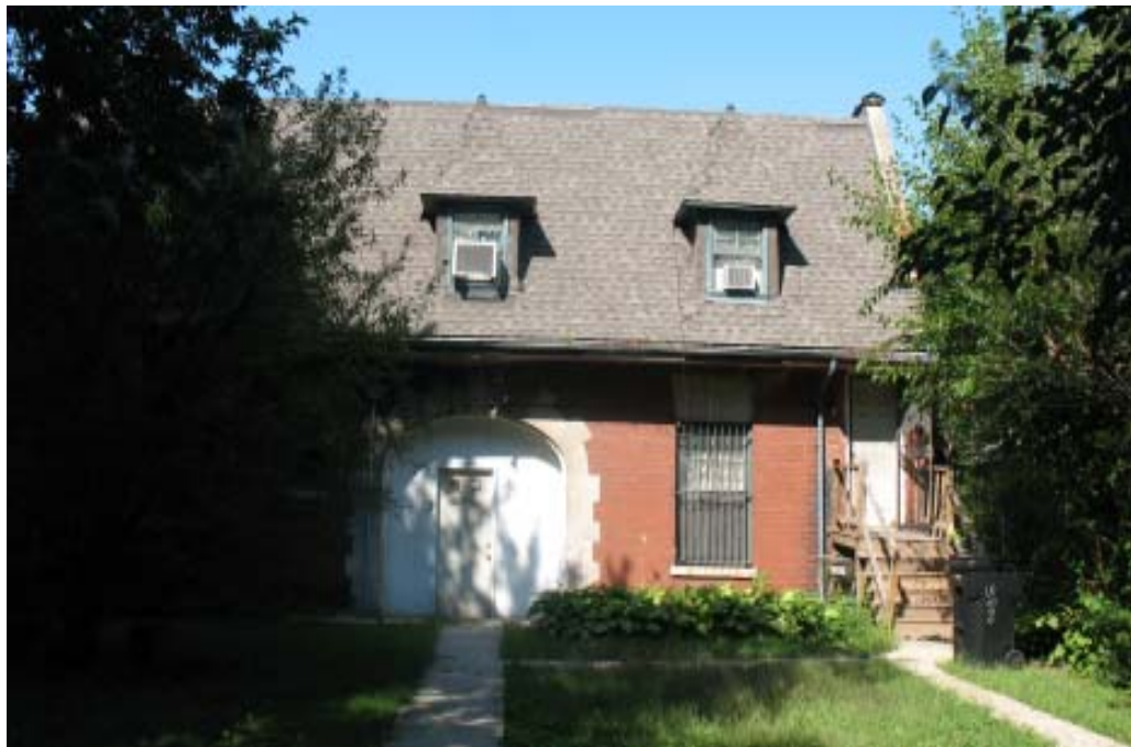
Top: A view of the house's north (side) elevation.
