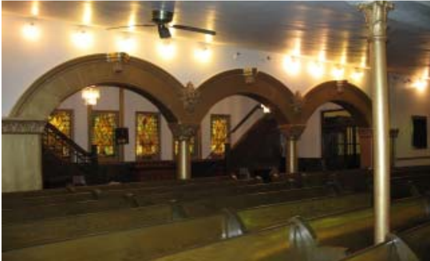
Top: The sanctuary is connected to an inner vestibule by a trio of round arches ornamented with Richardsonian Romanesque-style columns and capitals.
