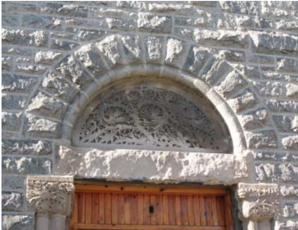
The exterior of the Kenwood United Church of Christ is ornamented with finely-carved stone columns and lunettes, detailed with Richardsonian Romanesque-style foliate ornament based on medieval ornament in Western Europe and the Byzantine Empire.
