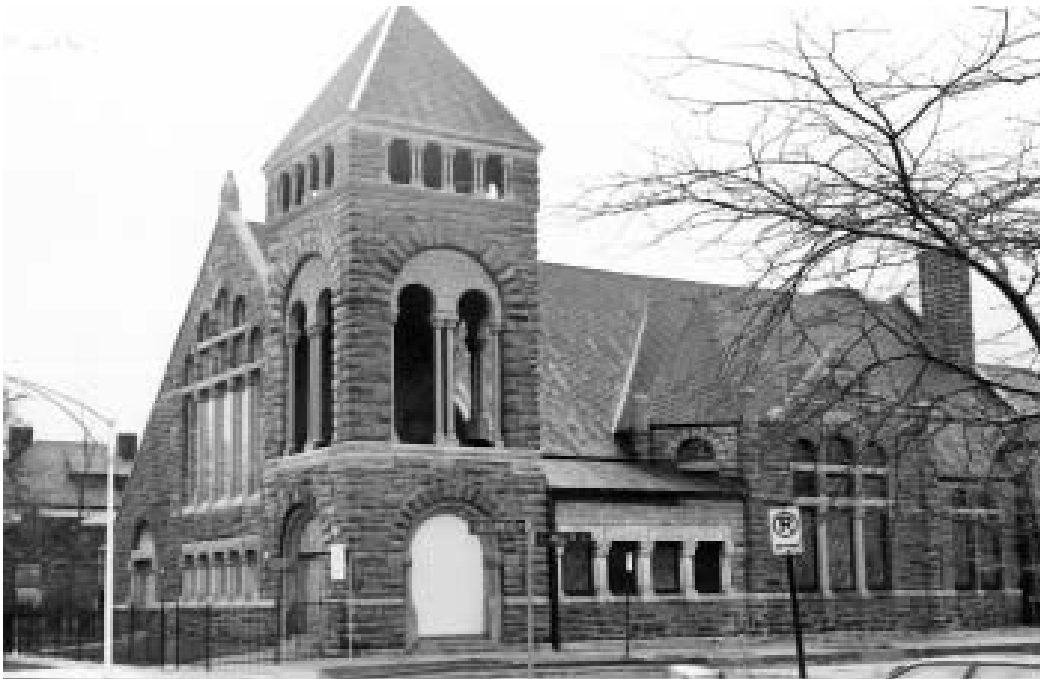
A photograph of the church building in 1991 when it was individually listed on the National Register of Historic Places. The building, including its rear Sunday school and gymnasium wings, is also located in the North Kenwood Chicago Landmark District.
