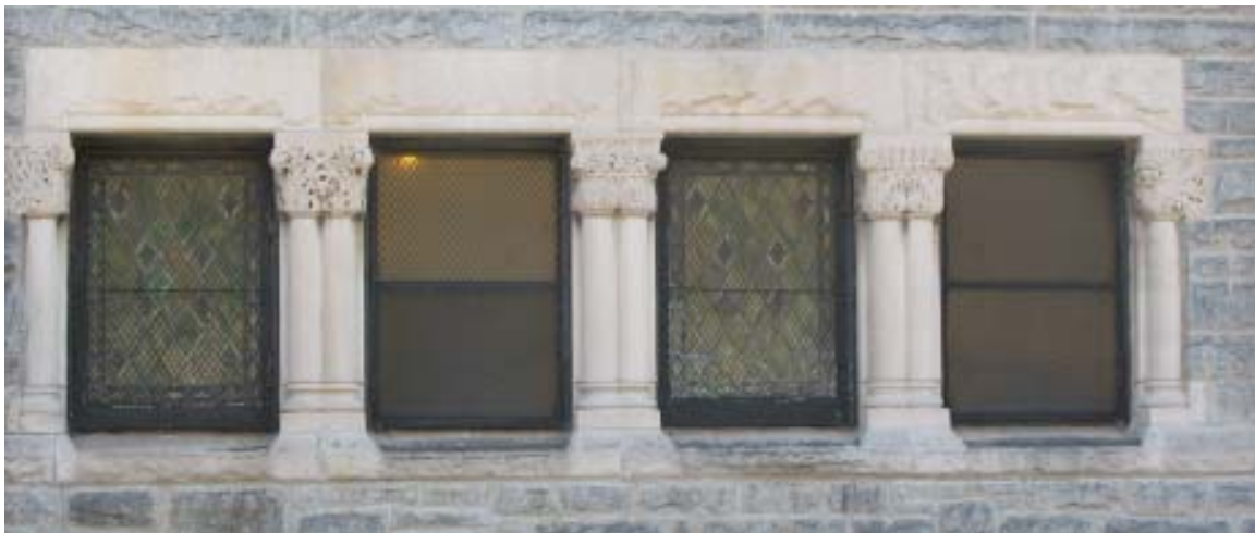
Exterior stone details of the Kenwood United Church of Christ, including (clockwise from top left) the corner bell tower, the foliate-detailed finial atop the front gable, foliate capitals, and a window row with paired columns with foliate capitals.
