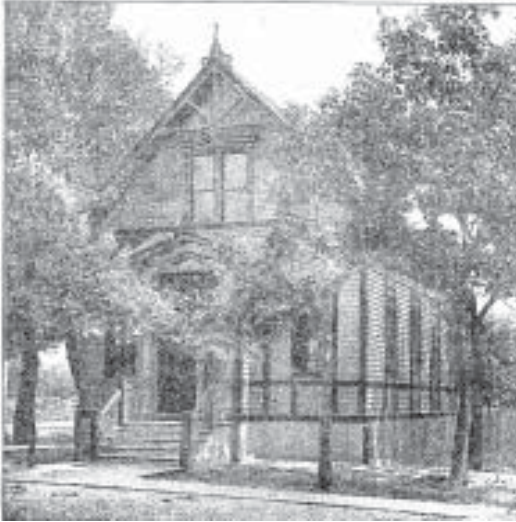
Left: The first home for the Kenwood Evangelical Church (as the Kenwood United Church of Christ was originally called) was a small wood-frame chapel located at S. Woodlawn Ave. and E. 44th St., south of S. Lake Park Ave.
