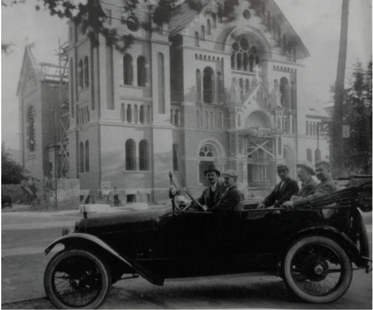
Historic photograph (dating from 1917) of the construction of St. Benedict Church on Irving Park Road. The gentleman in the rear seat closest to the photographer is Hermann J. Gaul, architect. Source unknown.
