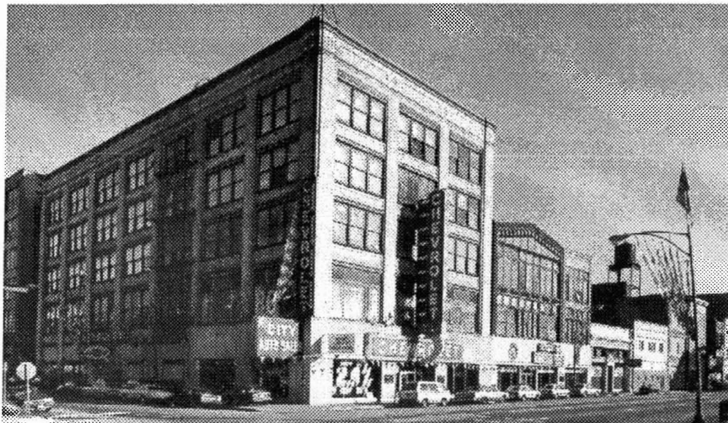
Auto-related buildings from 1910-15 grew even larger in scale as demonstrated by this group (above) at the southeast corner of 23 rd Street and Michigan for the Cadillac, Cowles, and Saxon showrooms (#35, 34, 33). An example of the layout of various departments (top) in such midrise structures was published in Motor Age magazine.
