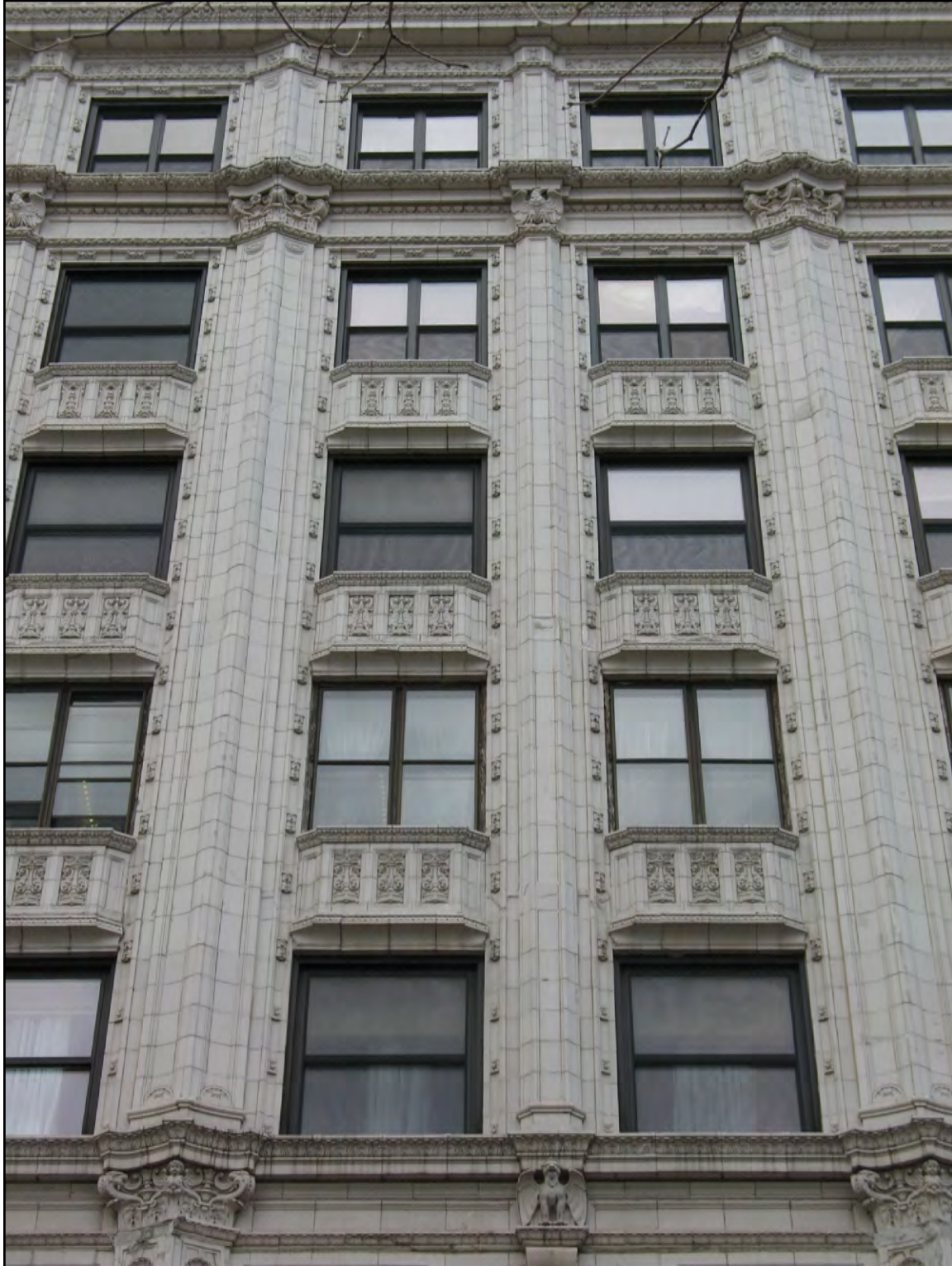
Opposite and this page: The Mutual Insurance Building's exterior terra-cotta facades are delicately ornamented with a variety of moldings and ornament used for cornices, window surrounds and spandrels.
