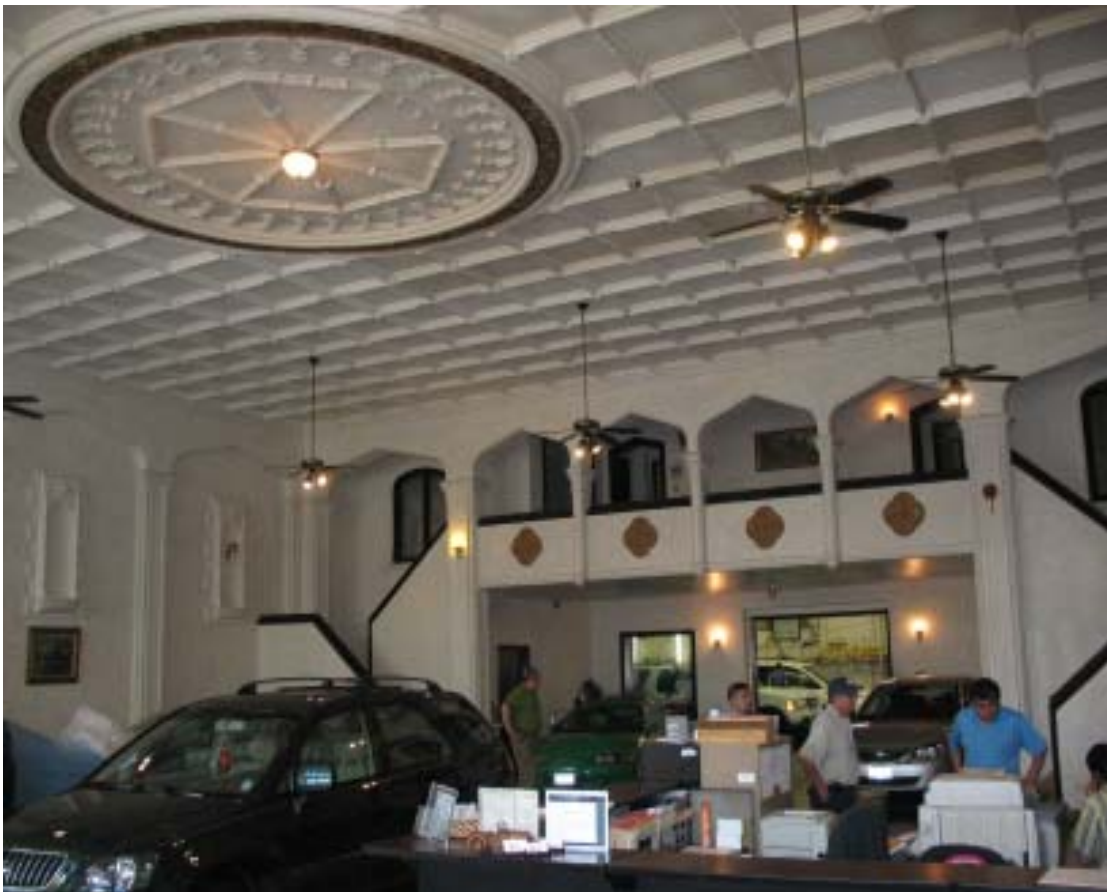
The Capitol Motor Sales Co. Building at 3041-43 W. Lawrence Ave. (1925-26) was also designed by R. Bernard Kurzon for the Burnstines. It is very similar to the Riviera Motor Sales Co. Building in its exterior terra-cotta ornament and recessed showroom entrance. Its elaborately-detailed showroom, with its high ceiling; shallow-grained plaster ceiling with tiny “bosses,” or decorative knobs; “blind” arches in the flanking walls, and open mezzanine reached by staircases also shares many similarities of materials and detailing with the showrooms in the Riviera Motor Sales Co. Building
