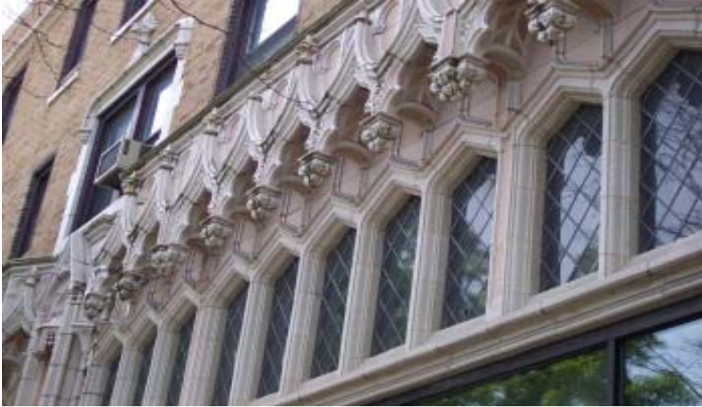
The Riviera Motor Sales Co. Building is detailed with lavish, finely-designed and crafted terra cotta ornamentation.
