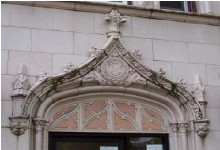
The Riviera Motor Sales Co. Building is detailed with lavish, finely-designed and crafted terra cotta ornamentation.
