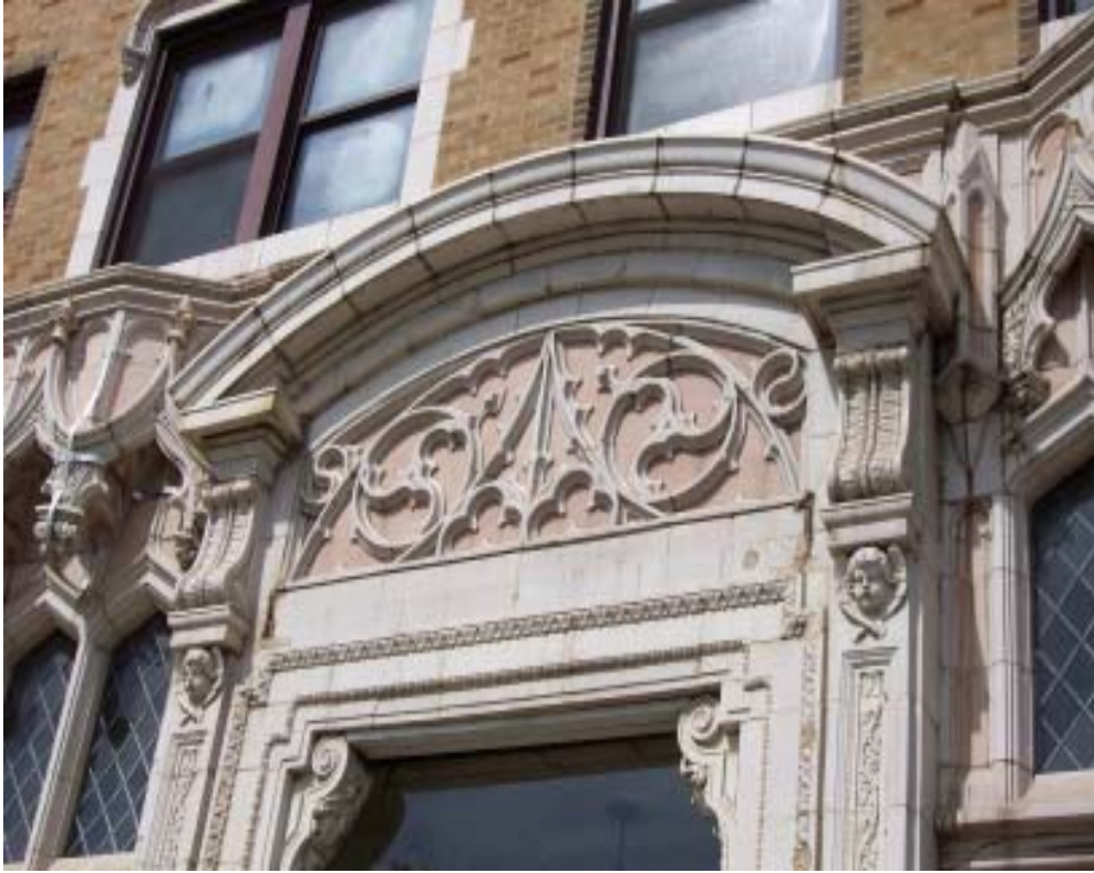
The Riviera Motor Sales Co. Building also has finely-molded Classical-style ornament around its two storefront entrances facing Broadway. Gothic-style “flame” tracery based on late French Flamboyant Gothic precedents is found within the round-arched pediment.
