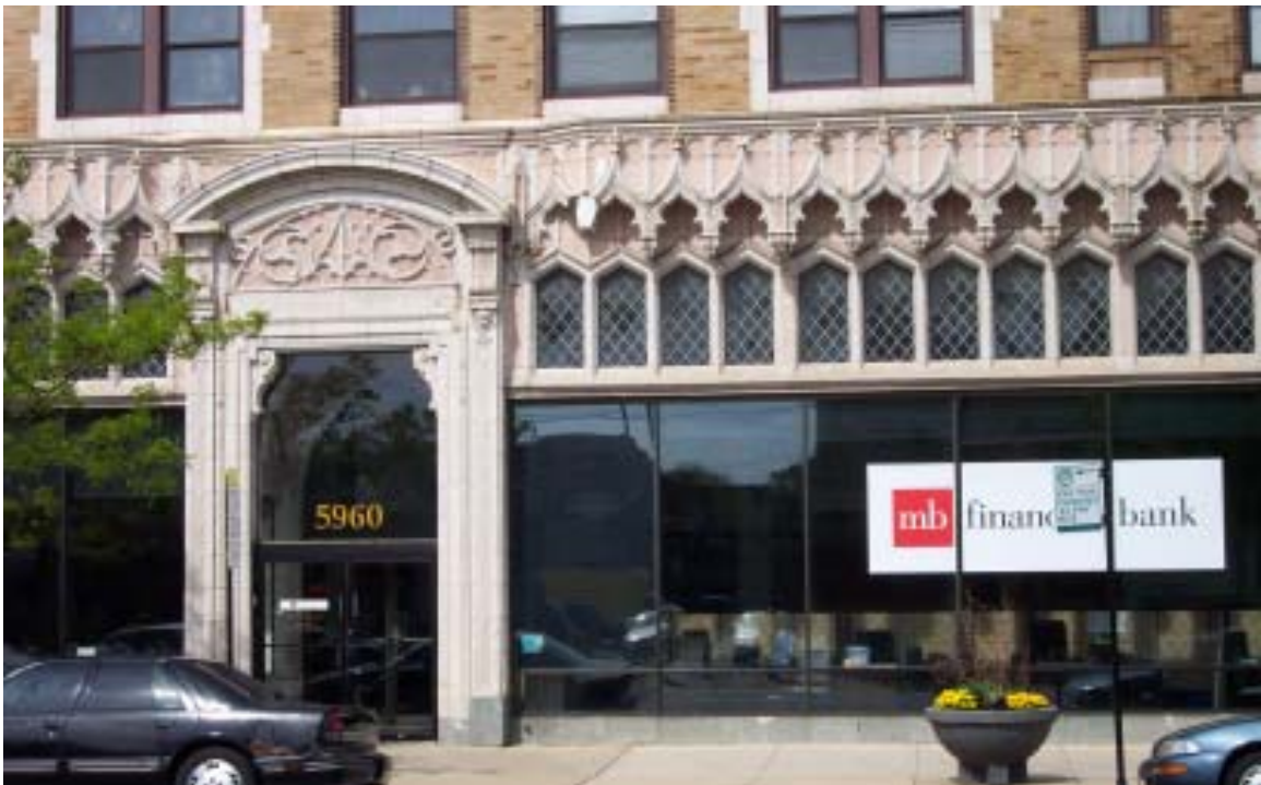
The Broadway elevation of the Riviera Motor Sales Company Building is visually dominated by the large glass storefront windows, terra-cotta detailing around the storefront entrances and especially the visually-lavish continuous decorative band above the storefronts comprised of boldly-molded Venetian Gothic-style hanging pendants and tracery.
