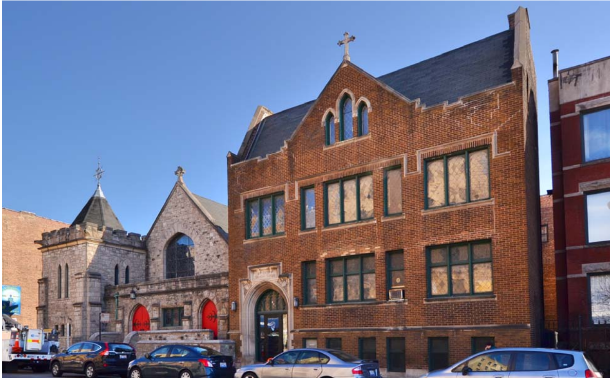
North elevation of the St. Peter's Episcopal Church and Parish House. The stone-fronted church ( left ) was completed in 1895, the brick parish house ( right ) was completed in 1926.
