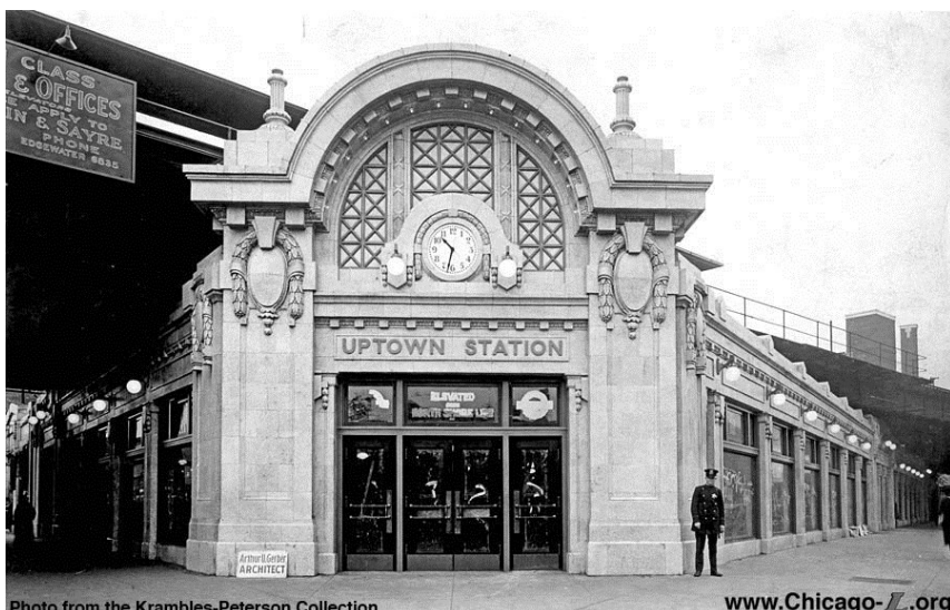
In 1922 the Stohr Arcade building was demolished to make way for the CTA Wilson L (Gerber Stationhouse) building designed by Arthur U. Gerber. A 2015 to 2018 construction project will provide exterior improvements and partially restore the building. Photo circa 1923.
