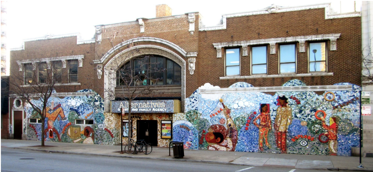
The Lakeside Theater (1914) adaptively repurposed as a community arts center.
