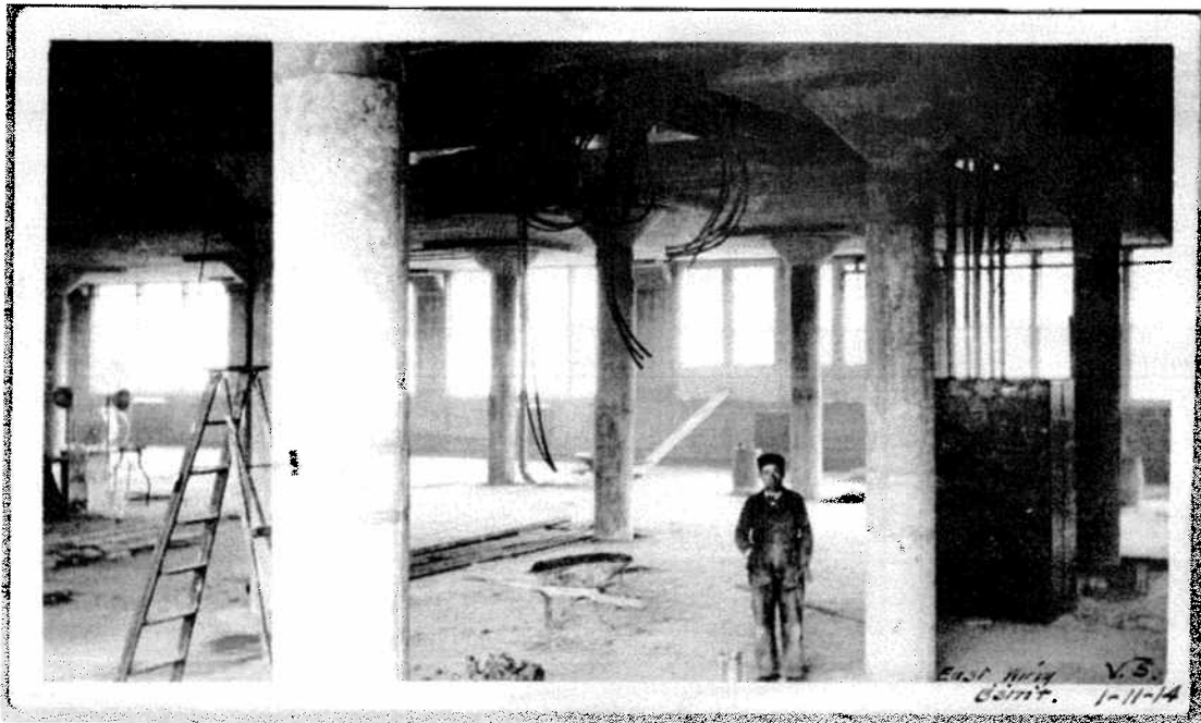
Construction of the original section of the Vassar Swiss Underwear Company Building begun in 1913. Above: The concrete structural system of the Vassar Swiss Building is clearly expressed on the exterior, forming a grid pattern whose concrete vertical members are the dominant visual element. Below: The interior was designed for optimum functional utility. Its concrete skeletal form employs the flat slab mushroom system variant, with vast expanses of large round columns topped with flared capitals. This system, with its flat ceiling uninterrupted by cross girders, allows for easy installation of unbroken mechanical conduit, pipes, and ducts.
