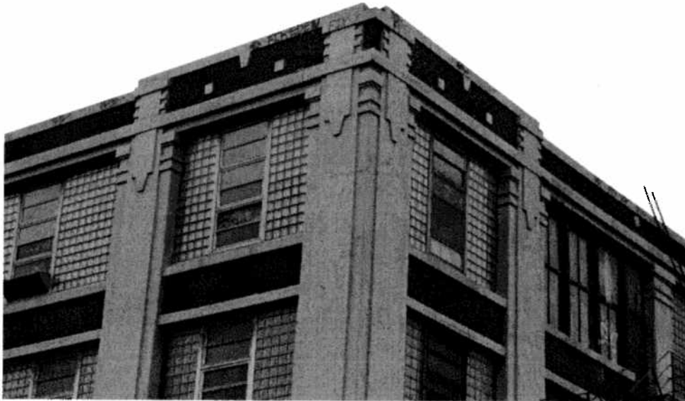
Exterior vertical concrete posts of the Vassar Swiss Underwear Company Building are treated as pilasters, with geometrically simplified bases and capitals. Window bays are separated horizontally by courses of “enameled” brick outlined with concrete sills. The corner bays of the structure have additional architectural detailing. These pilasters are wider, with Arts and Crafts-inspired capitals that pierce through the slightly elevated parapet. Small stone squares inset in brick further mark these corner bays. At the time of construction, the exterior concrete was reportedly given a second coat of concrete composed of marble dust and ground glass, to achieve a decorative white marble effect. Top: Diversey Avenue and Maplewood Avenue facades, photograph from 2007. Bottom: Corner detailing, photograph from 2007.
