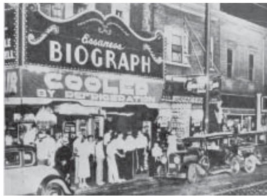
Above: The Village Theatre, ca. 1950s. The theater operated as the Gold Coast Theater from 1931 to 1962. The vertical sign was replaced with an awning-style marquee, similar to that of the Biograph Theater (right). Below: The marquee was again replaced with a prow-shaped marquee in the late 1960s.
