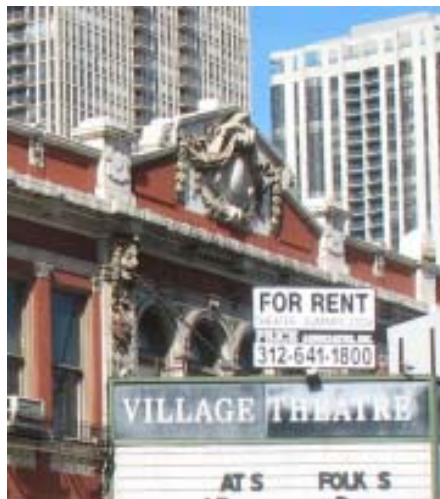
Above: A current view of the Village Theatre, designed in the Classical and Renaissance Revival architectural style. Middle: Above the theater's modern marquee are four round-arched windows (partially obscured). Below: One of the Village Theatre's storefronts retains its original window configuration, and a Classical Revival terra-cotta pediment denotes the deeply-recessed entrance alcove to the upstairs offices.
