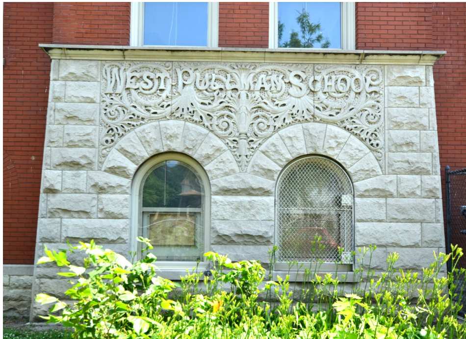
Left: Detail of stonework on the west bay of the 1894 building. The school name is set in raised letters against a foliate background. This design was copied and applied to the 1900 addition.
