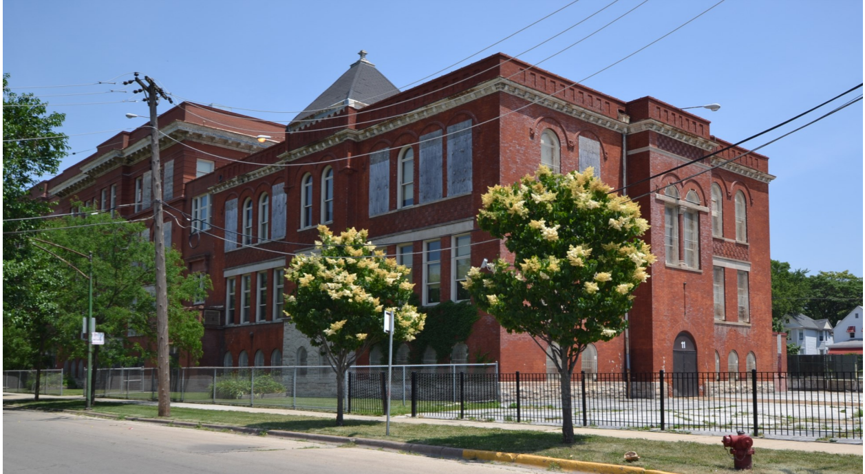
The original 1894 school building was designed by W. August Fiedler in the Romanesque Revival style, which features rich patterned brickwork, foliate stone and terra cotta, a dentiled metal cornice, and projecting bays. The west and south elevations are shown.
