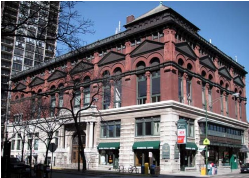
Left: Fiedler's Germania Club Building of 1889. The building is a designated Chicago Landmark.
