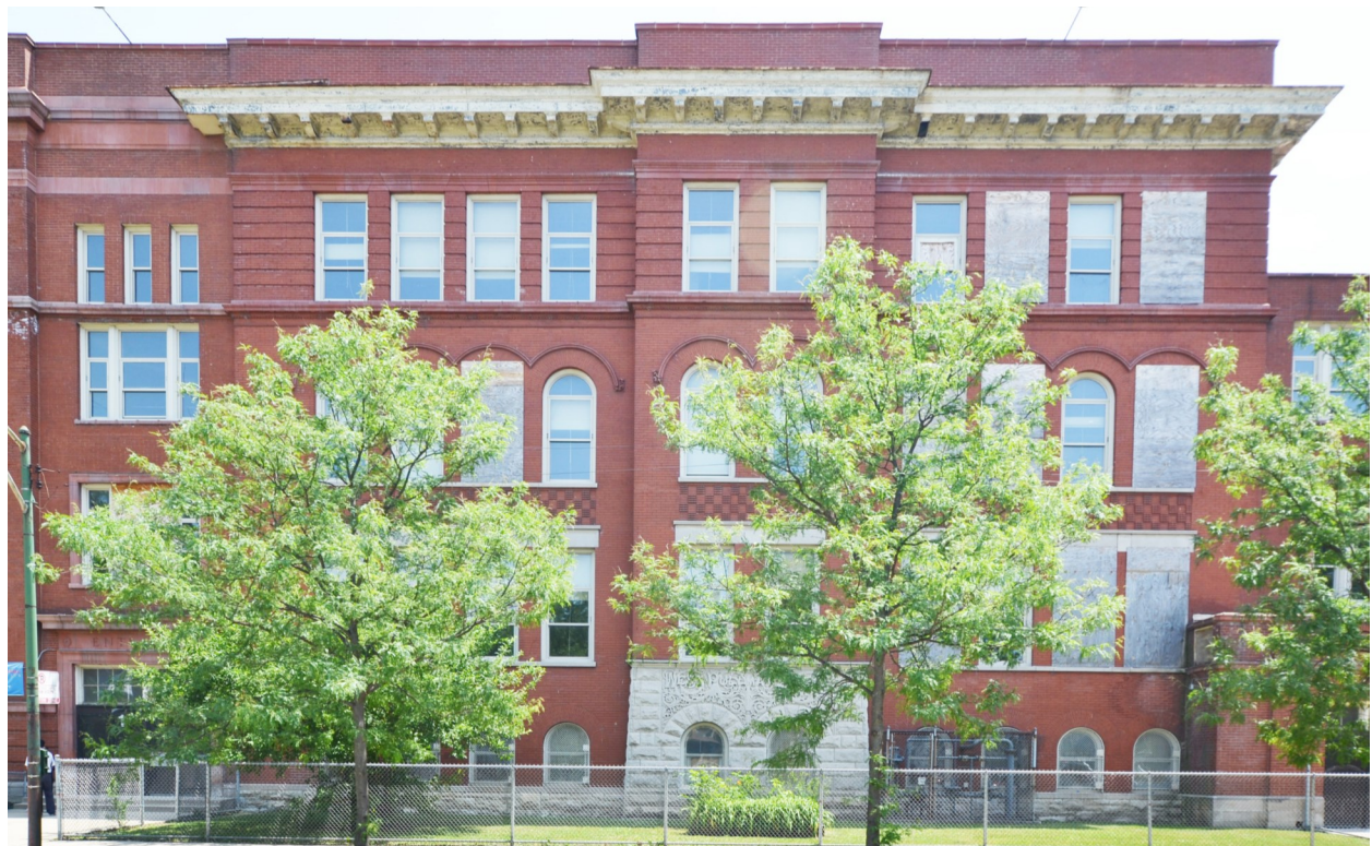
The 1900 addition was designed by William B. Mundie who retained Fiedler's original design for the first two floors of the addition, but added a third level in the Classical Revival style with rustic brickwork and a painted metal cornice. The west elevation is shown.
