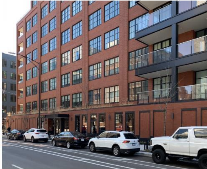
WASHINGTON BLVD. LOOKING EAST
