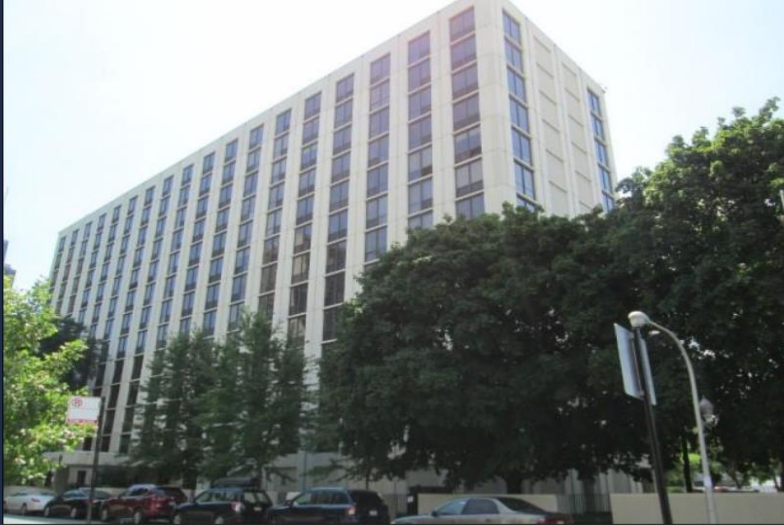
Front View facing southeast
