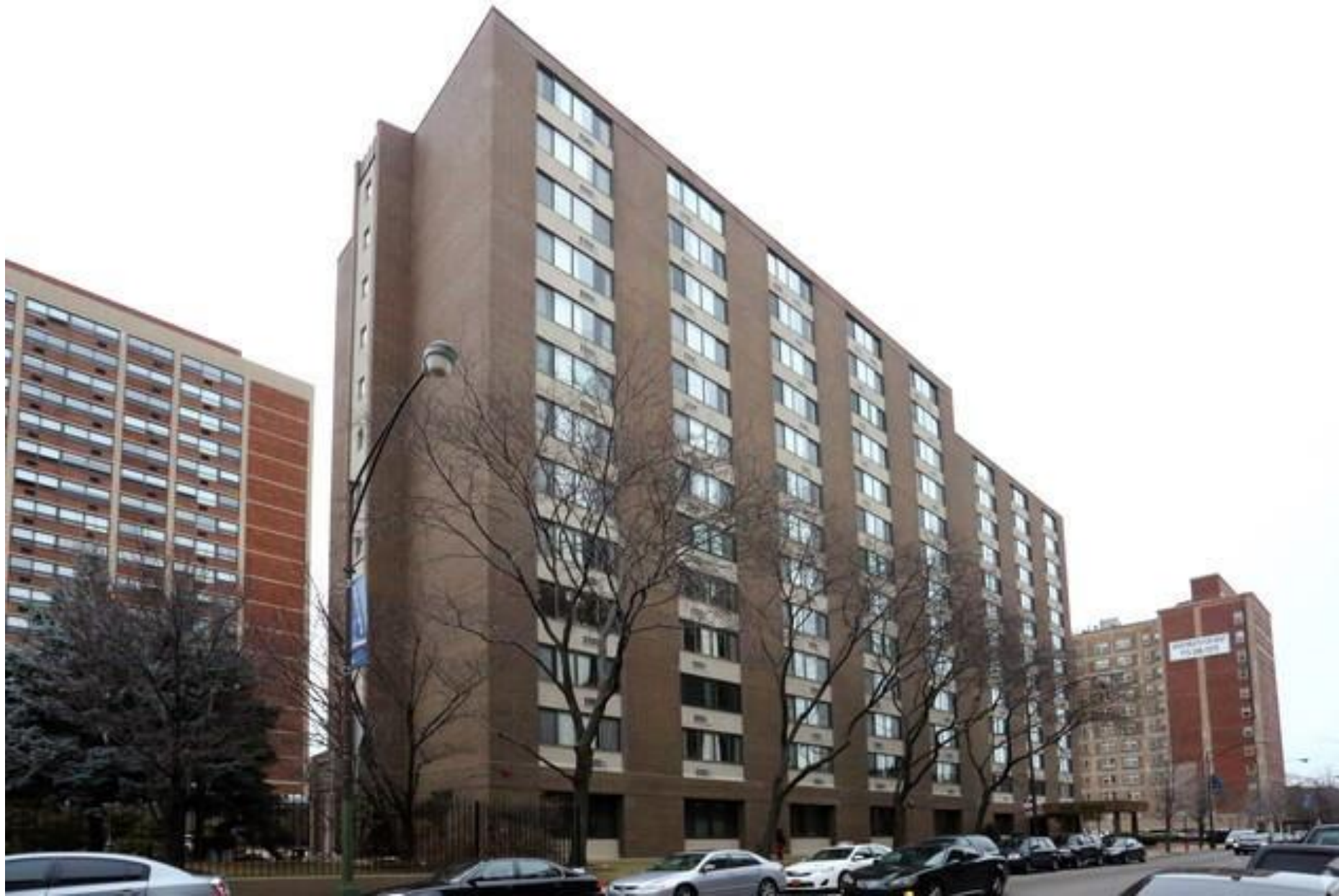
EXTERIOR VIEW – EXISTING CONDITIONS
