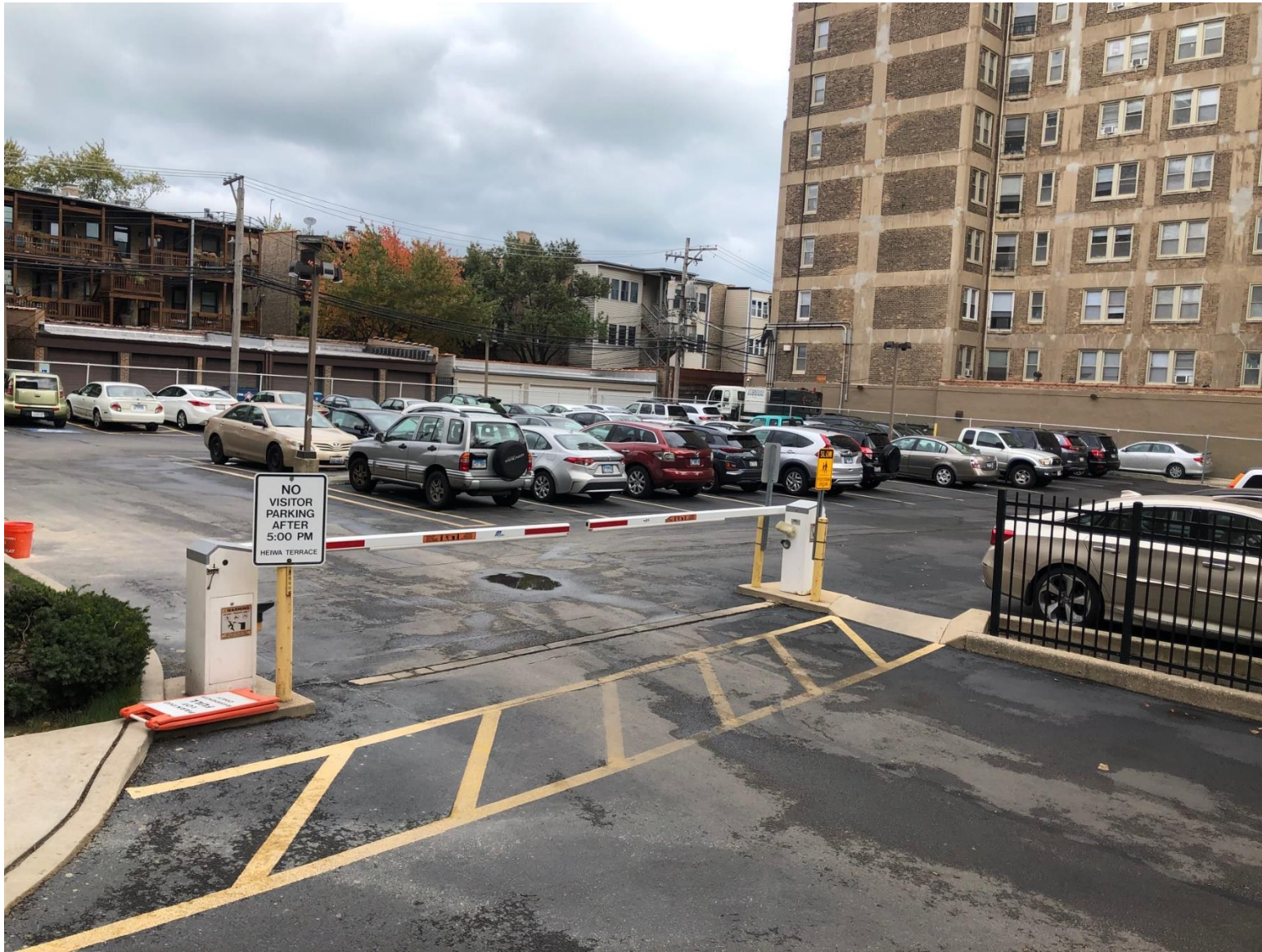
EXTERIOR VIEW – EXISTING PARKING LOT CONDITION
