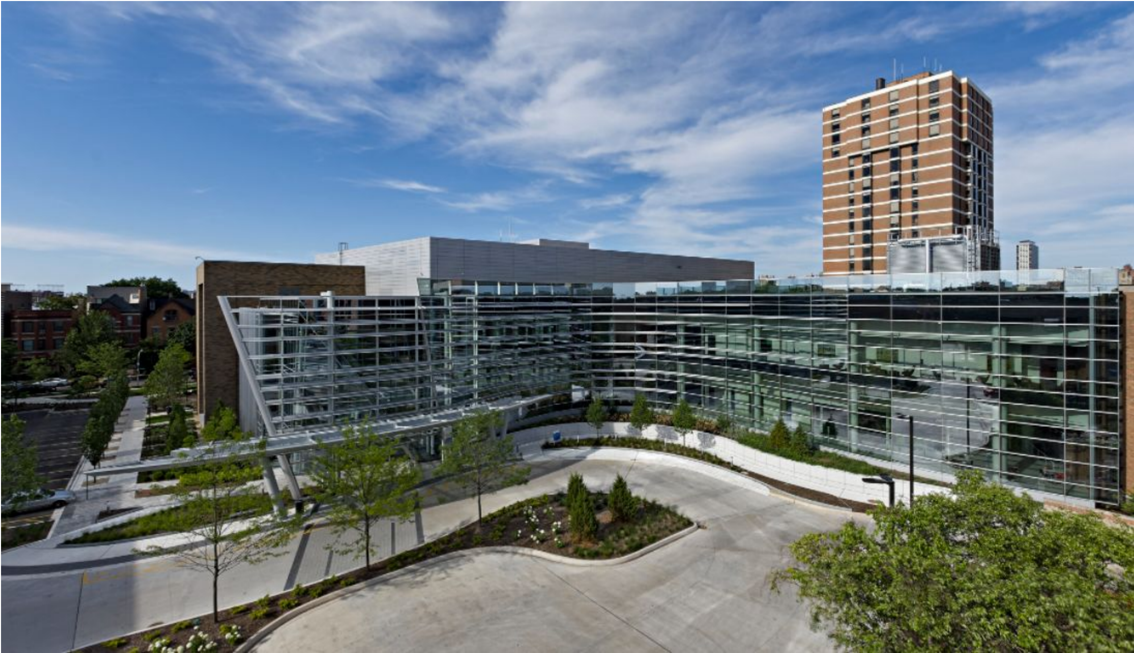
Vacated W. Nelson St. looking northeast
