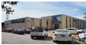
Toward the mid-to-late 20th century, new building materials were introduced such as, colorful glazed brick and metal or enamel panels. In the Kinzie Industrial Corridor, the building above is constructed of typical cream face brick accented by light bluish-grey metal panels.
