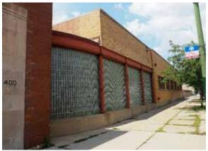
As steel became scarce during World War II many of the buildings constructed during this time in the Kinzie Industrial Corridor used glass block in lieu of the typical steel window.
