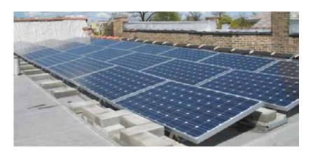
An example of a ballasted (non-penetrating) solar PV system. Here, the PV panels are not physically connected to the roof. Cinder blocks are used as ballasting means to secure the system to the roof.
