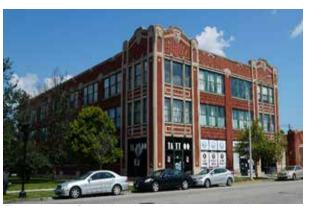
Typical use of traditional brick masonry with limestone ornamentation and detailing found in the Kinzie Industrial Corridor.
