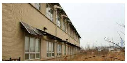
At the Chicago Center for Green Technology, solar panels serve a dual purpose, as they are used to generate electricity and are used as awnings above windows.
