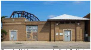
Example of brick masonry construction in the Kinzie Industrial Corridor with decorative inset terra cotta and limestone ornamentation at openings.
