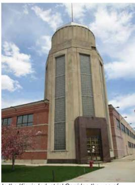
In the Kinzie Industrial Corridor, the use of limestone as building cladding and not only for ornamentation is rare. The tower portion of the building pictured above is only one of two examples of limestone cladding in the corridor.
