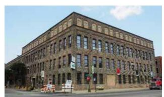
Historically, many of the buildings in the Kinzie Industrial Corridor were added to with one or two-story roof top additions. Pictured here is a typical example of a roof top addition (4th floor) in the Kinzie Industrial Corridor.
