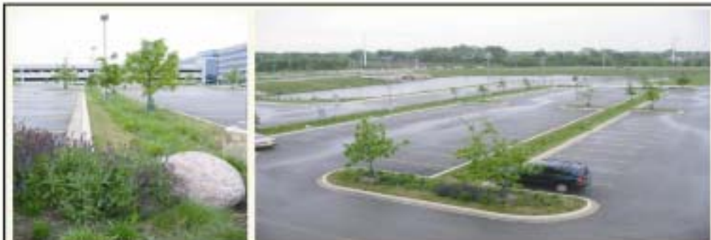
Parking Lot Bioswales
