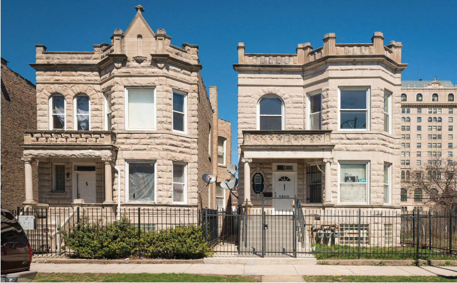
Chicago is home to many distinct building types, such as two-flat homes.
