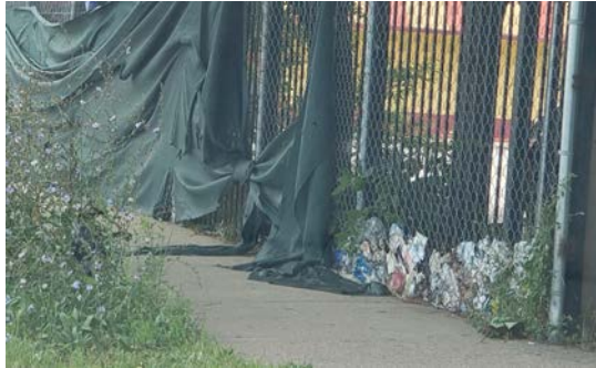
2020 Please address torn fence coverings and trash
