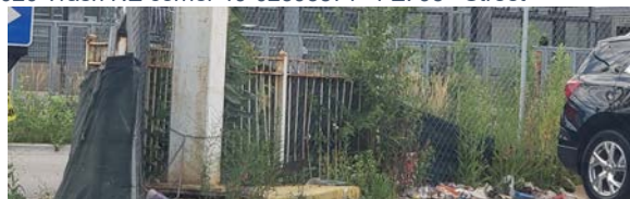
2020 Trash, torn fence covers. NE corner 4 E. 95th Street
