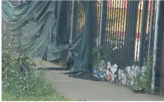
2020 Please address torn fence coverings and trash
