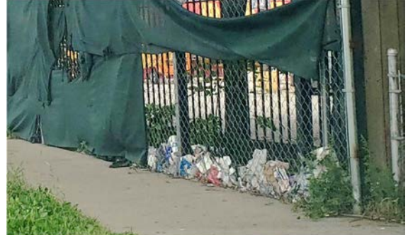
2019 Please address torn fence coverings and trash
